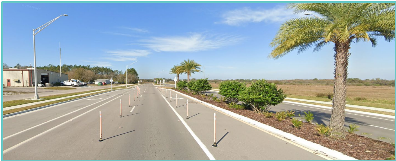
Figure 2-3 | Lorraine Road looking west at 44 th Avenue East
