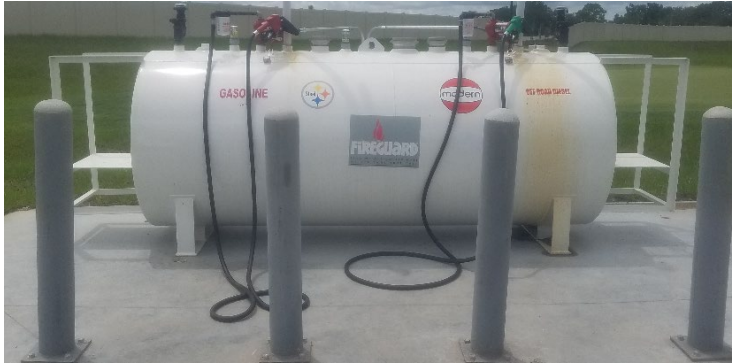
Figure 7 | Esplande at Azario Lakewood Ranch Golf Maintenance (FDEP Records 2020 Inspection)
