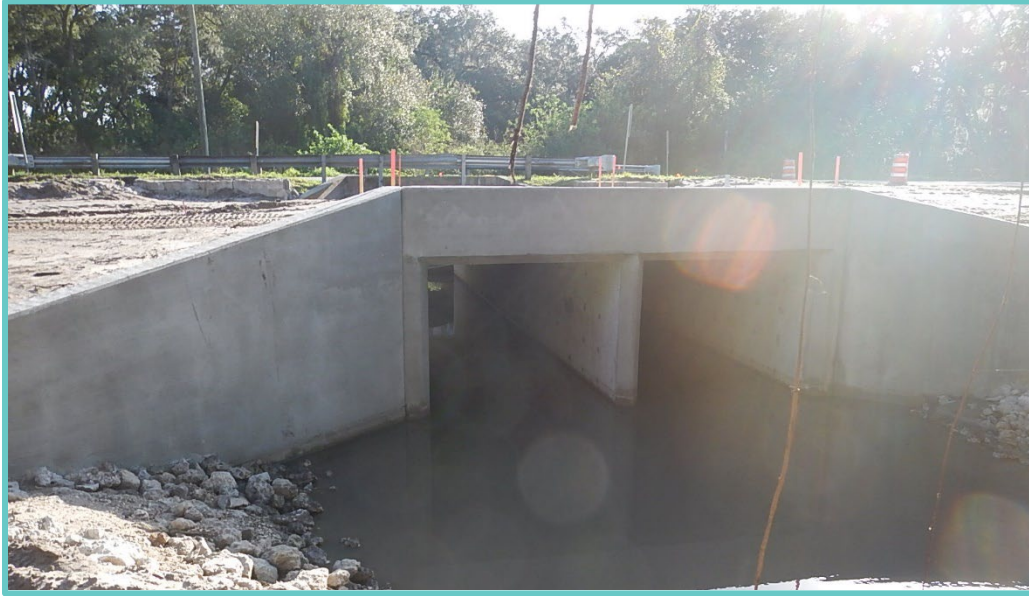
Figure 2-7 | Concrete Box Culvert NB2055
